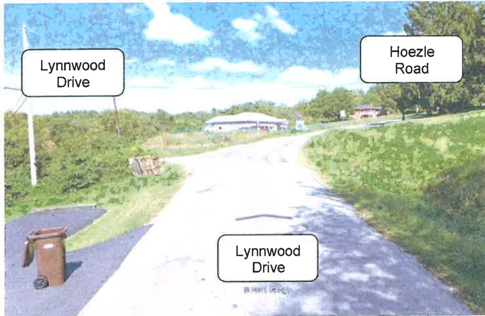
Figure 5: Lynnwood Drive Westbound approach looking at the intersection.
